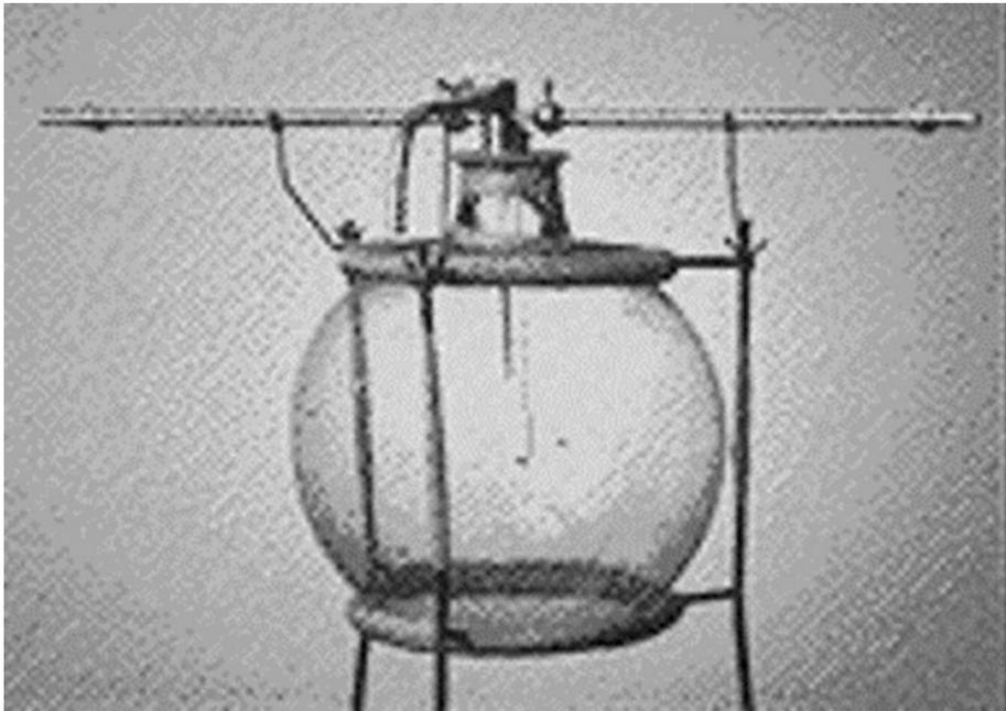
Figure 1-7 Lavoisier's apparatus for his hydrogen combustion experiment.
