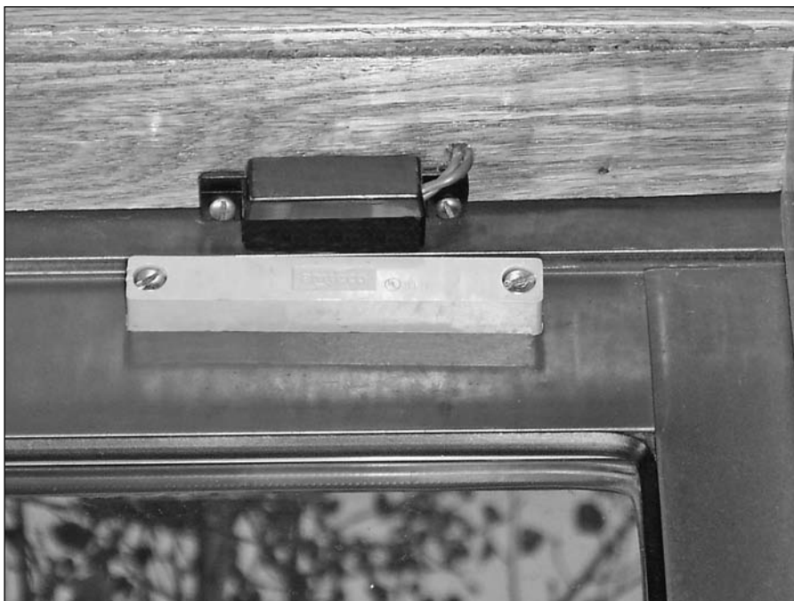
FIGURE 4-6: Magnetic door switch
